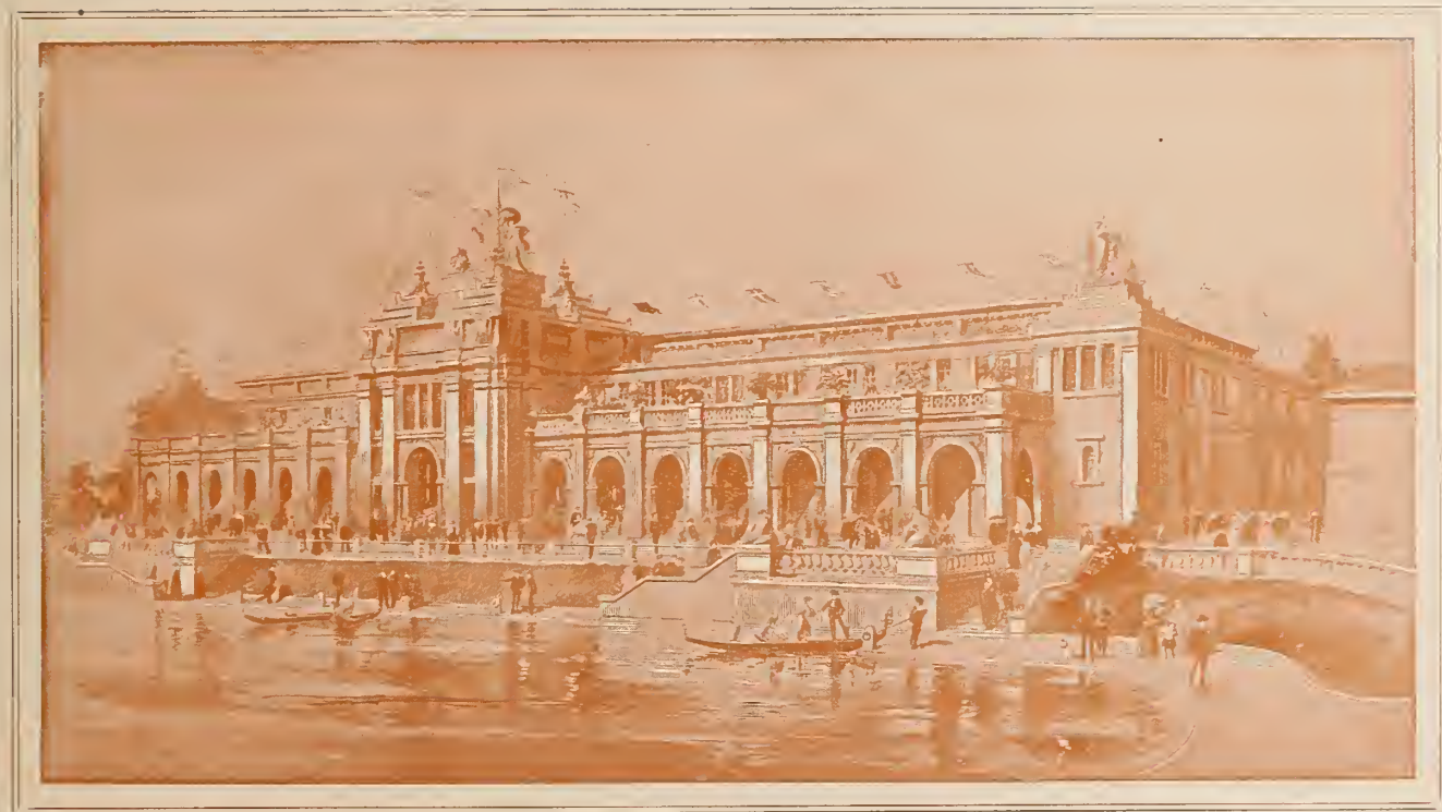
MACHINERY AND ELECTRICITY BUILDING.
